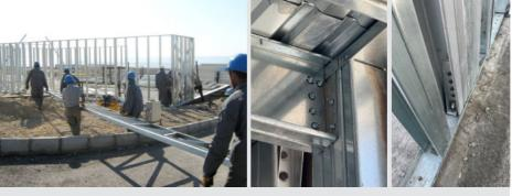
The steel framing is erected, anchored, and connected to the foundation and adjacent structural elements, ensuring proper alignment and stability. The panels are fixed through the use of hold downs, tie downs and chemical bolts.
