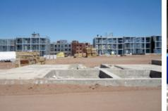
Excavation, levelling, and compaction of the foundation in preparation for LSF execution
