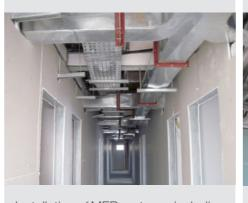
Installation of MEP systems, including electrical wiring, plumbing, heating, ventilation, and air conditioning.
