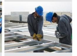
The fabricated components are assembled into panels according to the panelisation plan.
